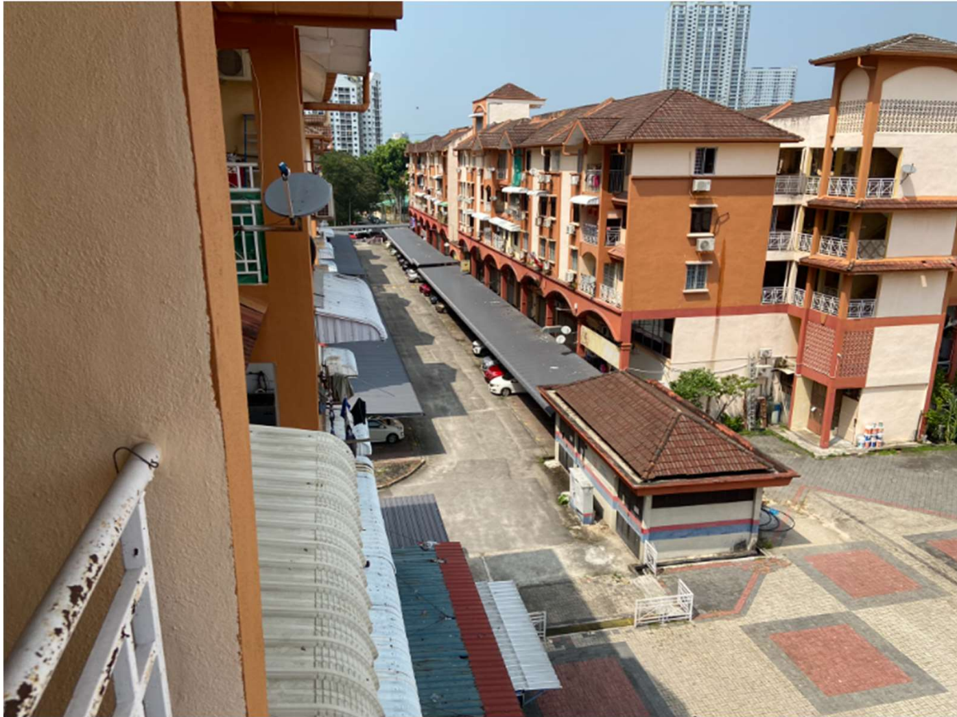
Individual car park which requires access card to enter and security guard at entry
